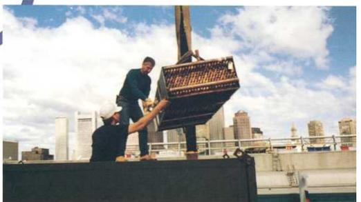
Technicians lower one of 16 custom made-to-fit replacement coils constructed by Heatcraft for Boston's World Trade Center. The coils had to be scheduled for delivery on Friday so that installation could be done when the convention center was empty.
